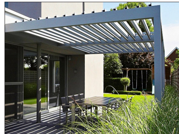
Cool cover: new roof system adapts to suit the weather
